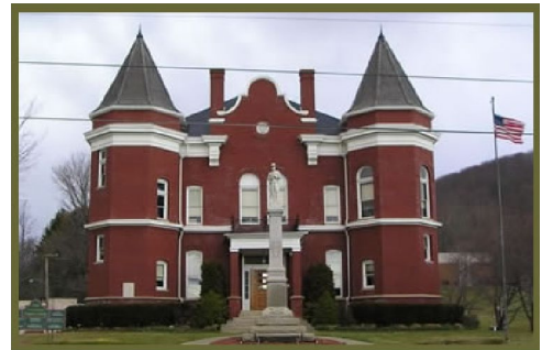
Figure 1-3: Historic 1908 Courthouse- Independence
